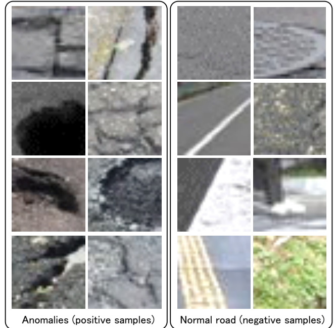
Fig. 5. Examples of local regions with anomalies or normal road surface for evaluating detection performance.
